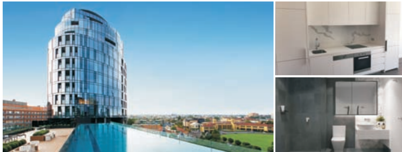
Project Name: The Parque City: Melbourne Solution: kitchen, vanity, laundry Qty: 329 units
