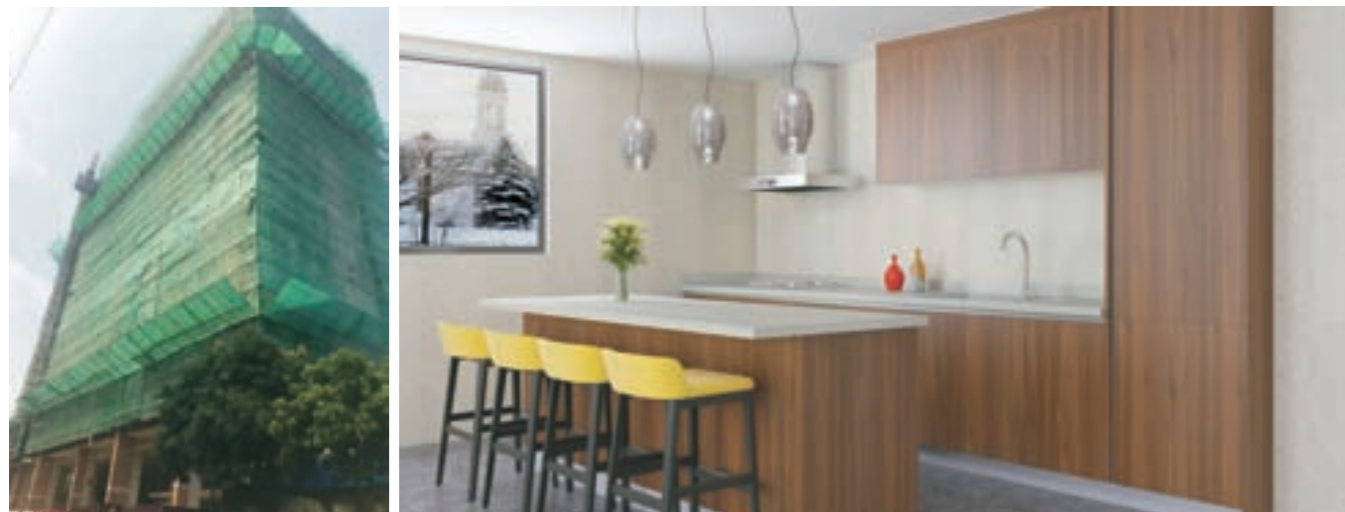
Project Name: KJKS APARTMENT City: Phnom Penh Solution: kitchen, wardrobes, TV cabinet Qty: 93 units
